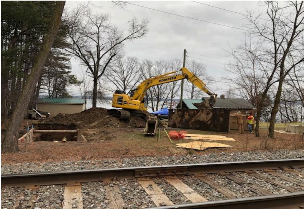
Contractor drilling under Railroad Tracks at North Serenity
