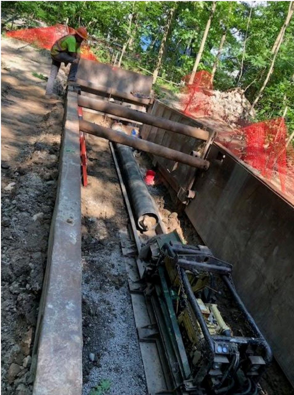
Bore being done on Caton Road
