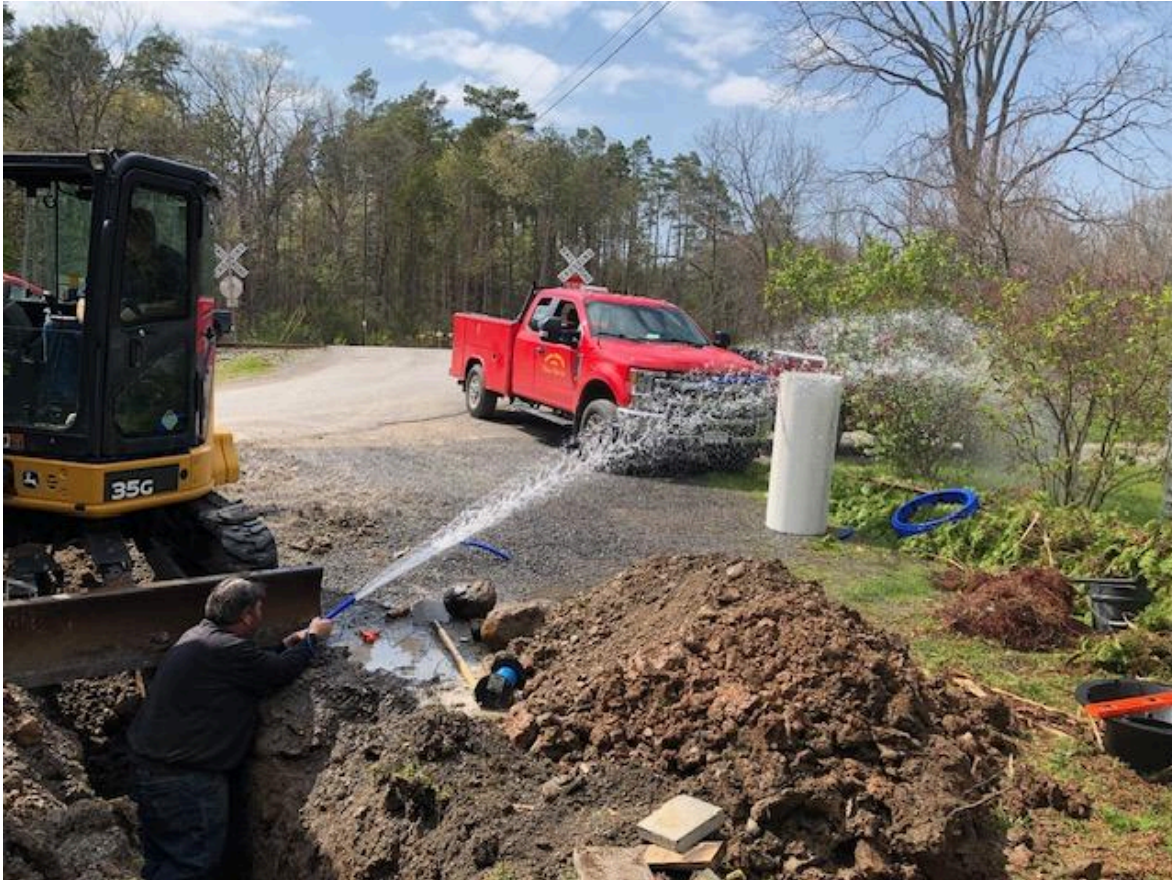
Tapping into the mainline on Serenity Road
